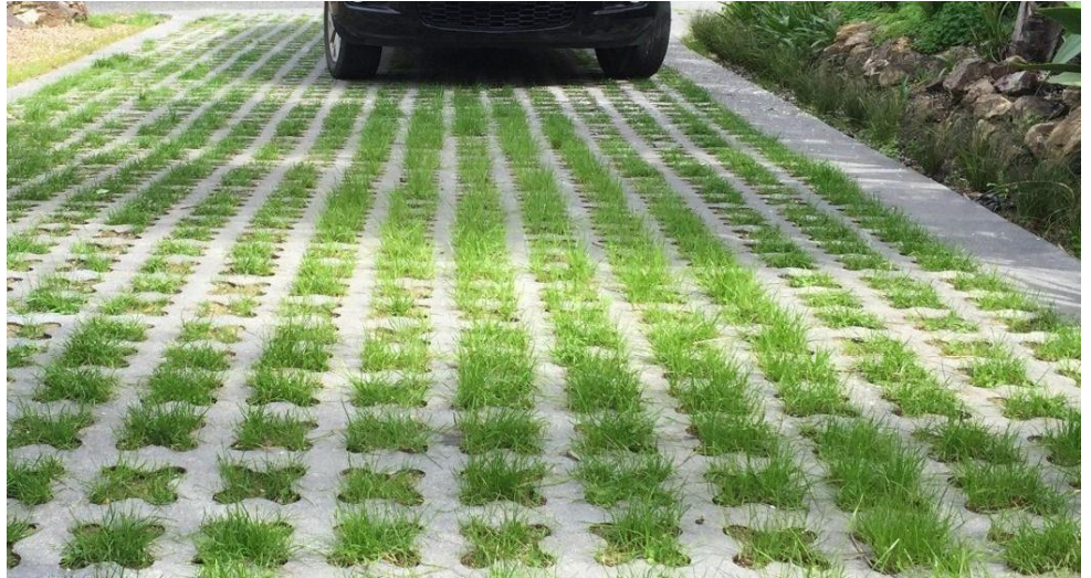
Figure 3: Example of installed indicative Grasscrete permeable paving system.
